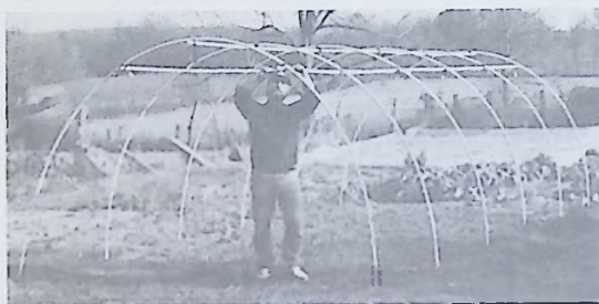
The nearly completed "hoop house" skeleton is prepared for the polyfilm cover, spread out in background. An inexpensive greenhouse can be made using 3/4-inch PVC piping spaced at four-foot intervals.
